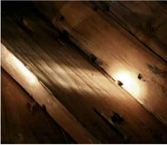
Side light is important for highlighting the relief created by tool marks. However, it can be difficult for the untrained eye to read and understand such traces. Photo: The Stave Church Preservation Programme 2002.
