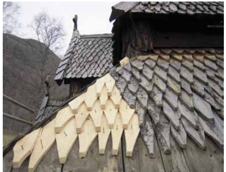
Replacing roof shingles; each shingle was fitted individually. Usable shingles were kept. There is no cardboard, foil or other waterproofing beneath the shingles. Photo: Harald Ibenholt 2009.
