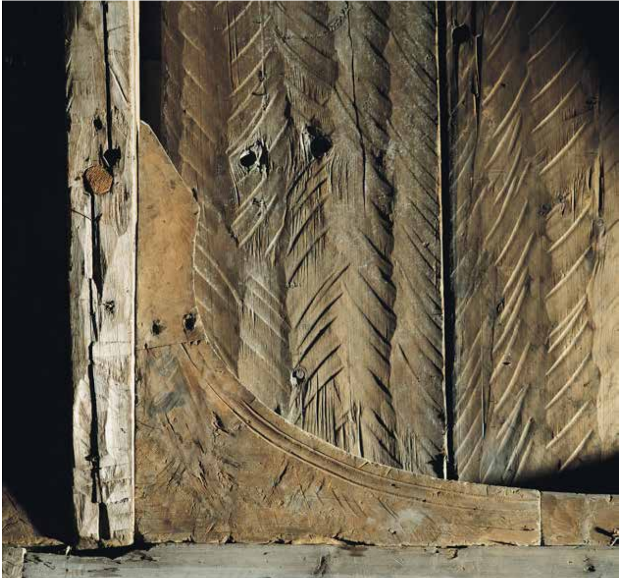
Section of the cladding in the ceiling of Haltdalen Stave Church. A wooden knee bracket binds together the rafter and the wall plate. Three by three vertical planks lie between the rafters. The ceiling has clear, marked traces of splash whittling. The axe marks are somewhat unusual as they run along the fibres. This cladding and the axe marks in the ceiling, are a good source for reconstructing the work behind the horizontal boards that lie above. Photo: Birger Lindstad 1999.
