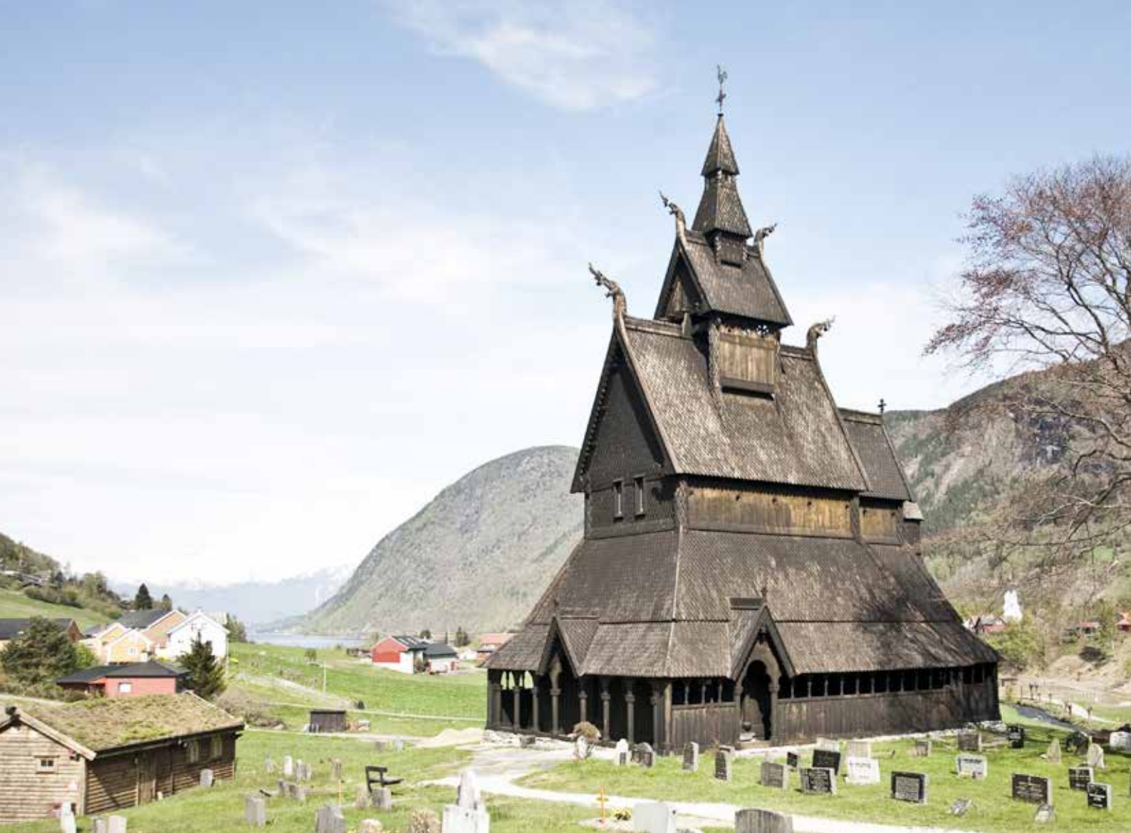
Hopperstad stave church, the roof was covered with sawn shingles during the restoration in the 1880s. Viewed from the south-west. Photo: Marcin Kaliński 2011.
