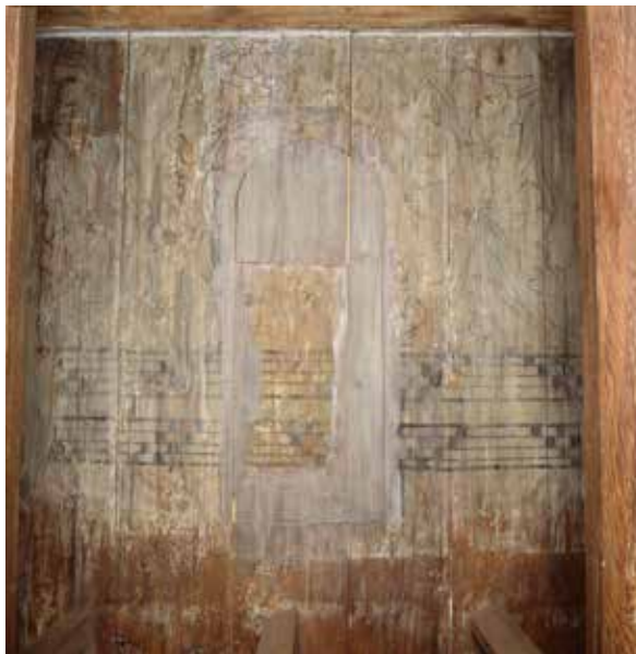
Kaupanger stave church. Part of the south wall with traces of a 1800s window inserted. The secondary inserted material is muted using a grey-white «wash» with oil-based paint. The original colourful decorative distemper painting has been reduced to a weak, almost black and white decoration. Below the vines in the nave is a vertical frieze of neums, a musical notation from the Middle Ages. Photo: Birger Lindstad 2008.
