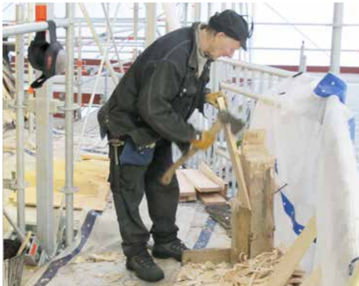
Axel Andersen hewing new shingles at Borgund. The photo was taken on the scaffolding. Photo: Sjur Mehlum 2011.
