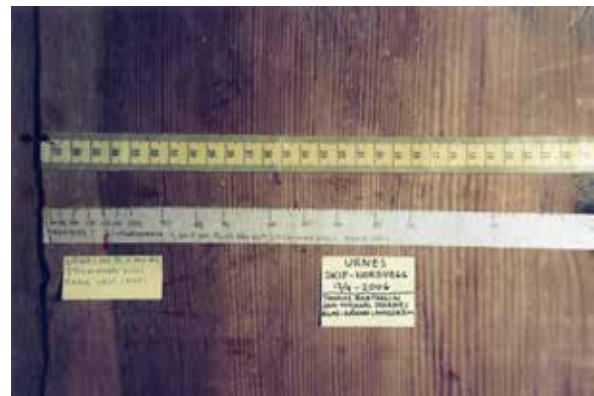
III. 13. Uppermost in the picture of plank no. 15 from the east, the sapwood has been preserved and the outermost tree ring is from 1069: this is the youngest dated tree ring for the north wall.
