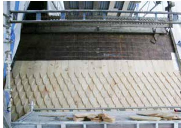
Replacing roof shingles at Hopperstad. Unlike Borgund, here the shingles were changed in whole areas. There is no cardboard, foil or other waterproofing beneath the shingles here either. Photo: Nedre Jølster bilelag, undated.
