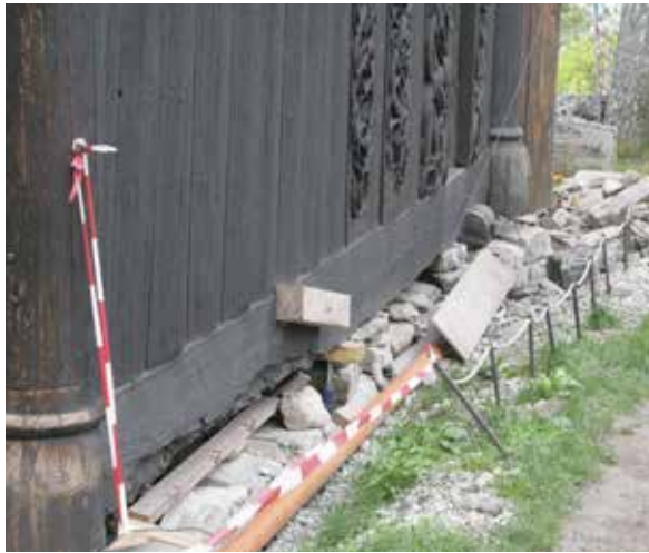
Rot-damaged sill beam on the north wall of the nave. The foundations were repaired, but not the rotten material, as it is not load-bearing. Photo: Sjur Mehlum 2009.
