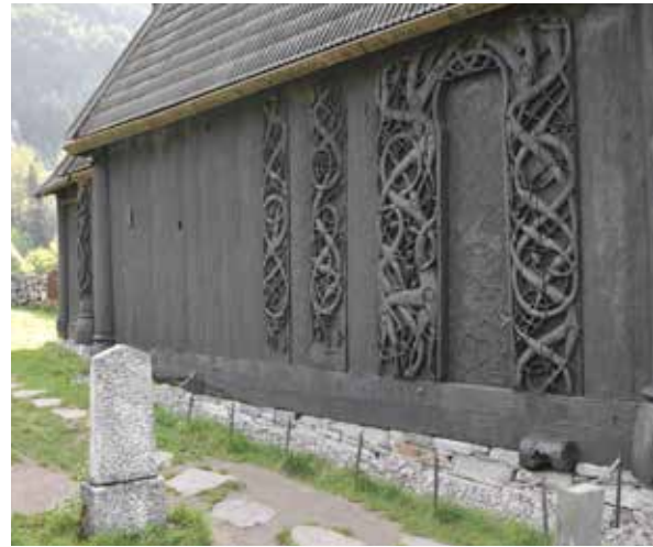
New foundations under the sill beam on the north wall. The sill has been raised by about 10 cm with good clearance from the ground. This will help prevent further rot damage. Photo: Leif Anker 2013.
