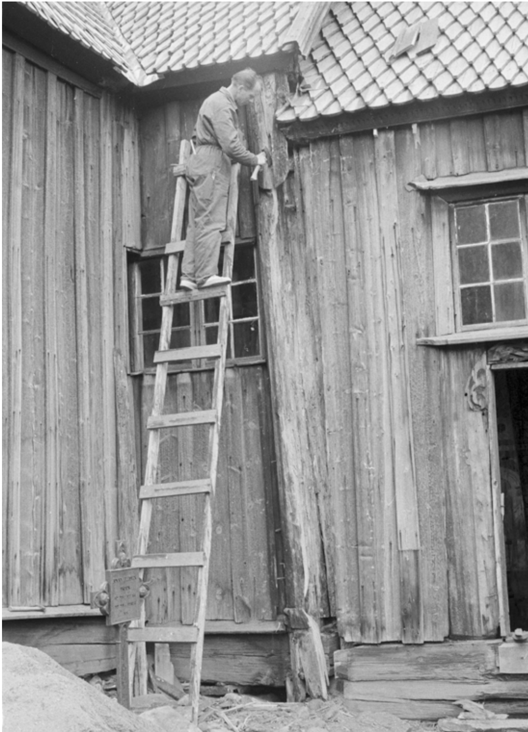
Nore Stave Church. South-east corner post of the nave has extensive rot damage along the whole length of the post. It was also repaired in 1969. Photo: Arne Madsen 1969.
