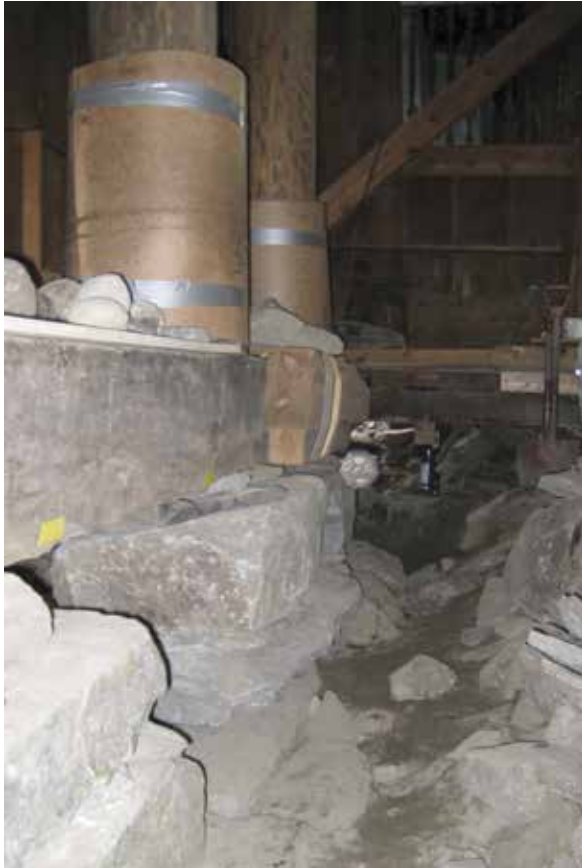
New foundations under the raft beams, work done during the Stave Church Preservation Programme. Photo: Marit Westli Arntzen 2009.
