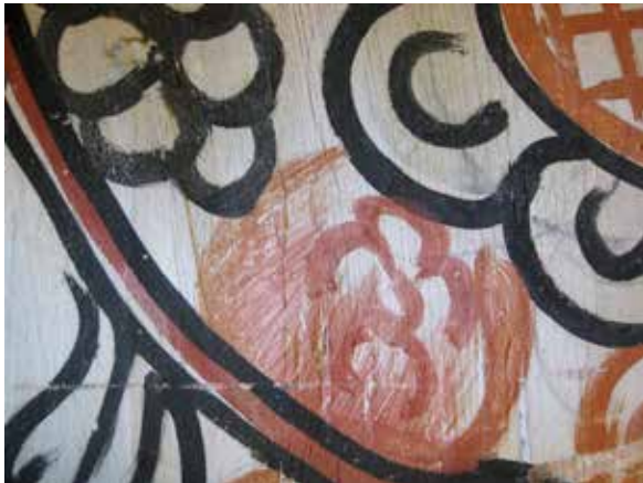
Umes stave church. Detail from the vine decoration from 1601 on the north wall. The decoration is drawn on a thin, white ground with a silver-coloured hard pen which can be seen in the upper-right of the picture. Then the coloured areas are painted: blue, red and a yellow-red. Finally the black contours are painted which define the motif. As is the case here, there is often little correspondence between the sketch and the final contours. The sketch appears to have been done to place the motif on the wall. This could be interpreted as the painter knowing the motif he wants to paint, or that he has a model. Photo: Tone Marie Olstad 2011.
