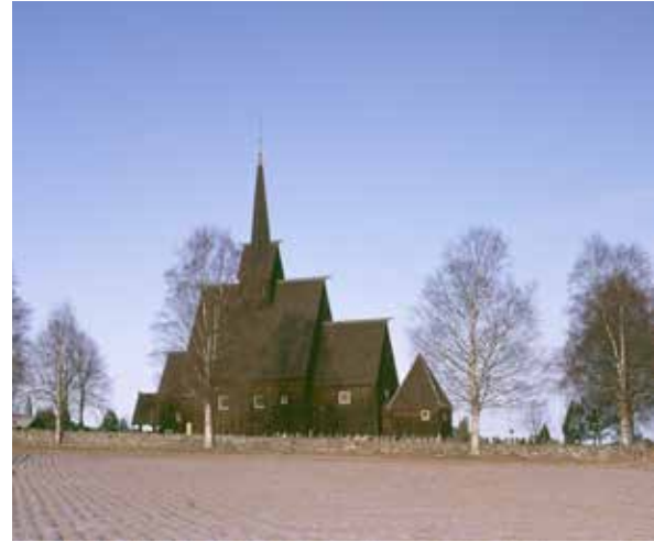
Høyjord stave church after the extensive interior and exterior restoration, completed in 1953. The roof became steeper, with a new tower and a tall spire supported by a central mast. The panel cladding is new, and old window openings have been re-installed with lead glass. Photo: Birger Linstad, Riksantikvaren.
