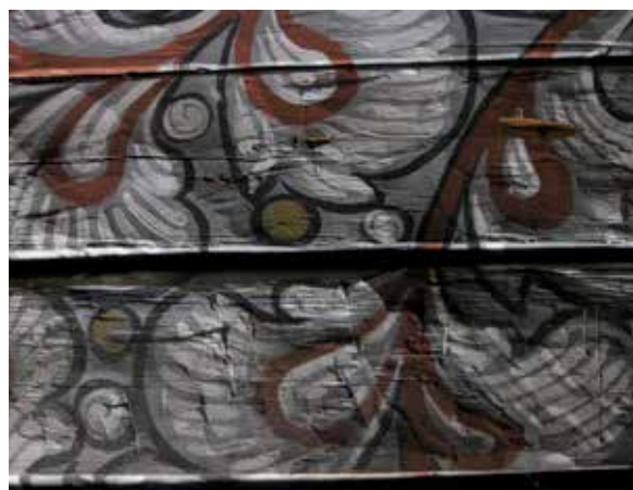
Nore stavkirke. The decorative distemper painting was painted directly onto the hewn surface and no further working of the wooden surface was needed. Here the vines on the timber walls of the southern gallery at Nore can be seen. These resemble the vines in the nave's oldest ceiling, but are freer and more coarsely painted. This adornment was probably added just after 1709. Photo: Tone Marie Olstad, undated.
