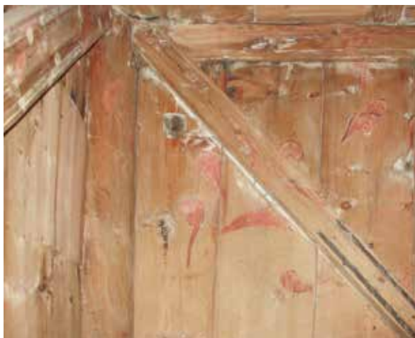
Borgund stave church. Good lighting reveals traces of decorative distemper painting in a number of places in the washed church interior. Here fragments of vine decoration can be seen up on the wall in the south-east corner of the nave. The colours in the wood show the direction of the vines. Photo: Tone Marie Olstad 2015.
