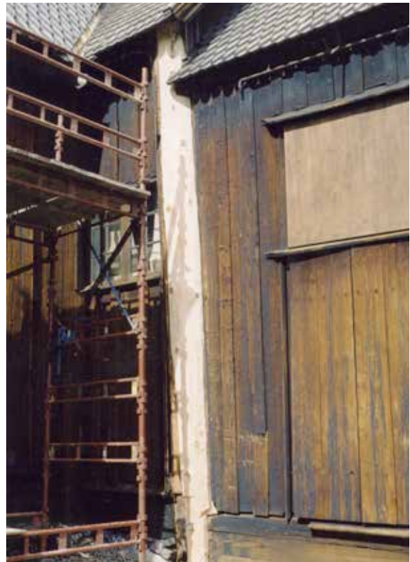
Repaired south-eastern corner post. The post was then panelled as it was before repair work commenced. Photo: Hans Marumsrud 2003.
